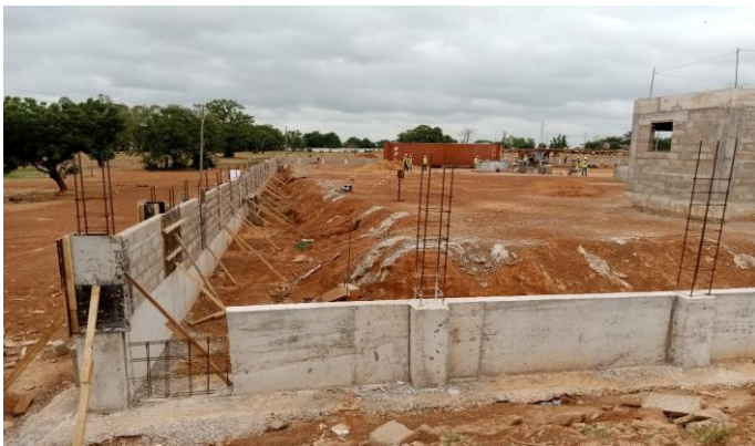
Lamashegu North Boundary Fence wall.
