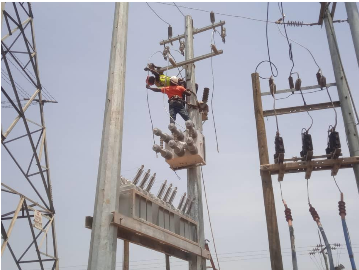
Installation of Capacitor Banks and drop out fuses.
