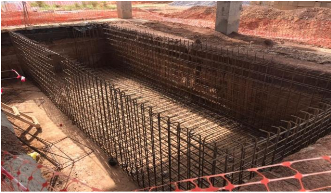
Adubiyili Switchgear Cable trench rebar installation.
