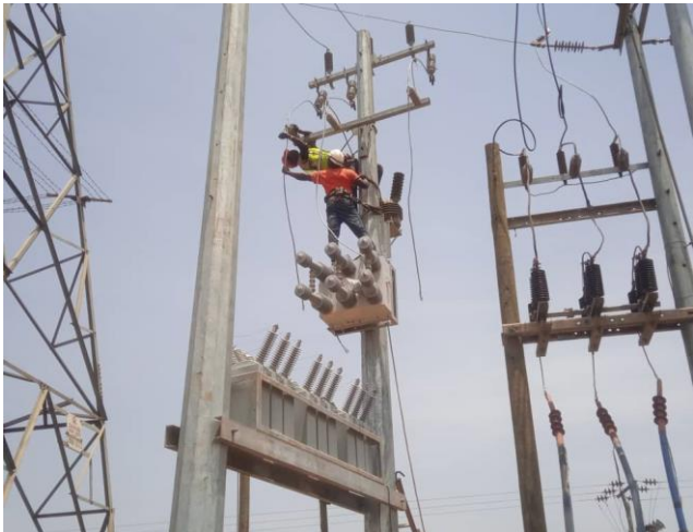
Installation of Capacitor Banks and drop out fuses
