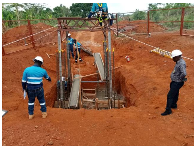
Construction of Tower Foundation
