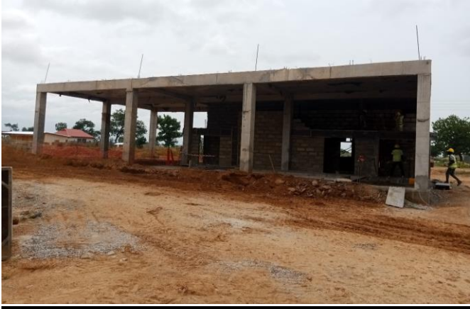
Back view of Adubiyili Control building
