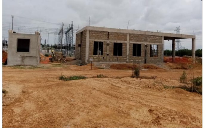
Front view of Adubiyili Security Gate house and Control Building.
