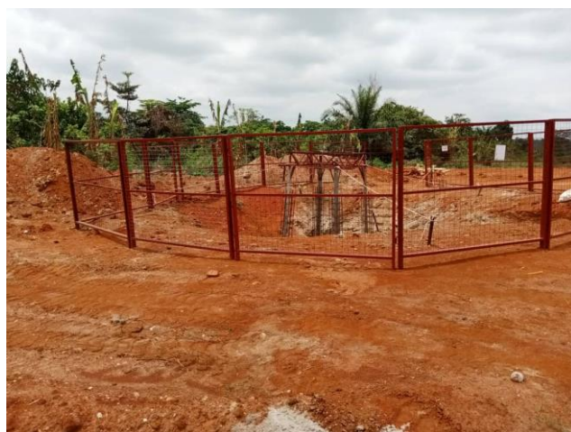
Construction of Tower Foundation
