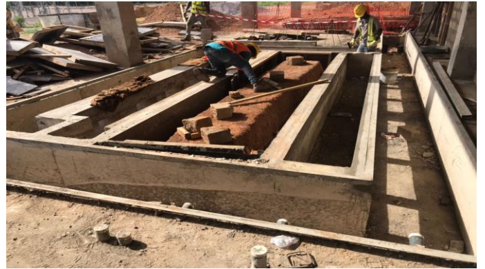
Adubiyili Control building communication cable trench concrete works.
