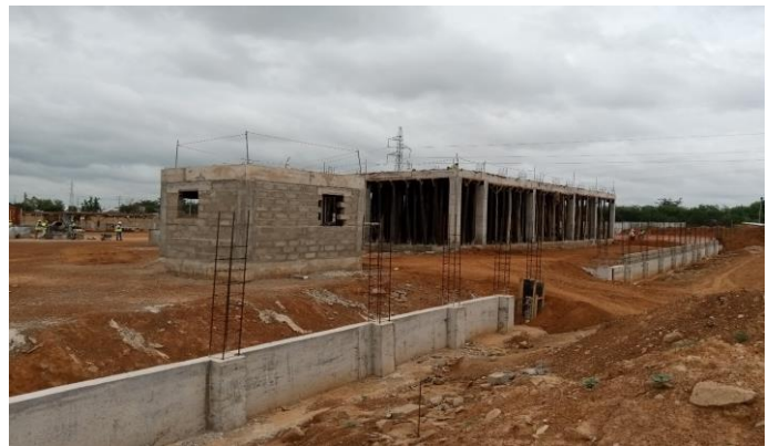
Lamashegu West Boundary Fence wall.
