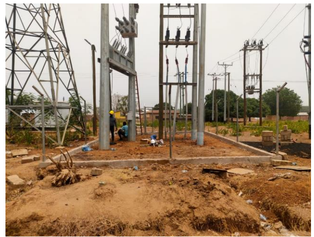
Preparation of Ground works and Fencing works
